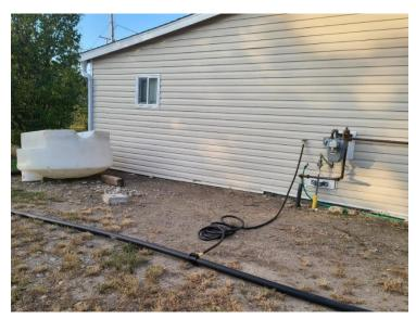
Temporary piping should not block any lanes, driveways or streets throughout the duration of construction. Where required, temporary ramps constructed of granular material, timber or other suitable material will be constructed to provide access.
