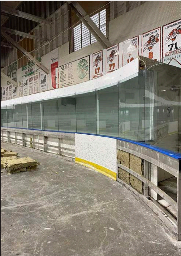
Puck Board and Board Frame replacement and repair.
