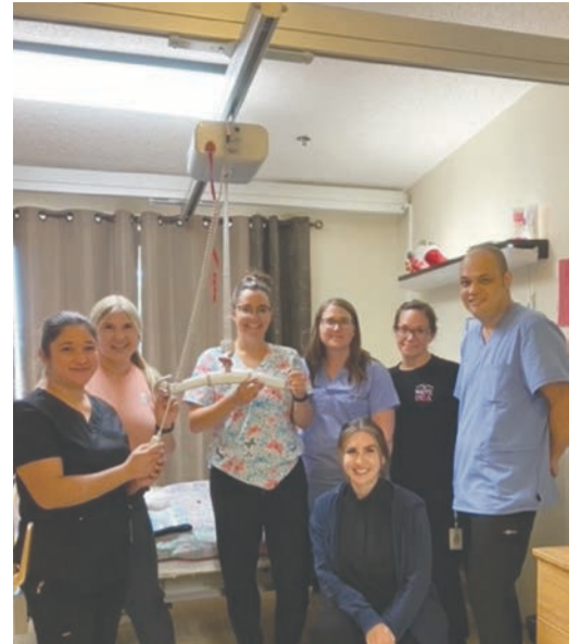
NEW TRACK LIFT Residents & Staff at the Heritage Manor are very thankful for the ceiling lift that was recently installed thanks to Ladies Night Out - 2022. Committee members Robin Bowden, Candy Gordon, Chelsea Omness & Joanne Kosolofski would like to thank all our sponsors & volunteers for their continued support. October 21, 2023 is set for Ladies Night Out. SUBMITTED PHOTO
