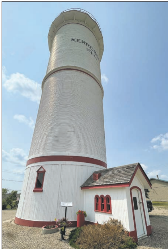
This standpipe reservoir in Kerrobert was built in 1914 and is one of three of its kind remaining. It is located next to the Kerrobert golf clubhouse.
