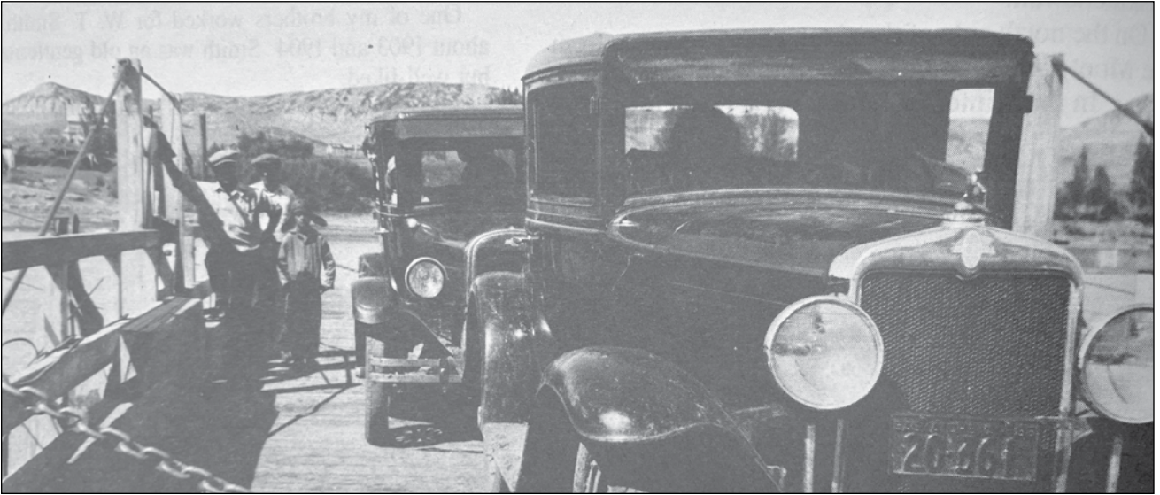
PRELATE FERRY IN 1933: Sometimes it was necessary for travellers to drive in water to meet the Leader Ferry at a sand bar. PHOTOS FROM A PAST TO CHERISH
