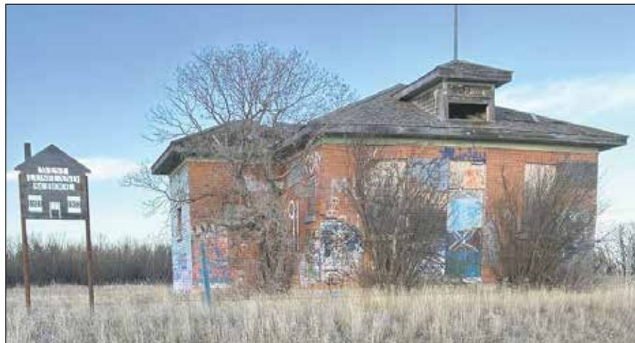
Luseland Museum shared some exciting news last week with the installation of the Country School signs! The work was completed by Travis Kasas at Carl's Mobile Welding and look fantastic! This photo is of the West Luseland School. Thanks to Kennedy's, McKenzie's, Reiter's and Holton's for their help with the installation. PHOTO LUSELAND & DISTRICT MUSEUM
