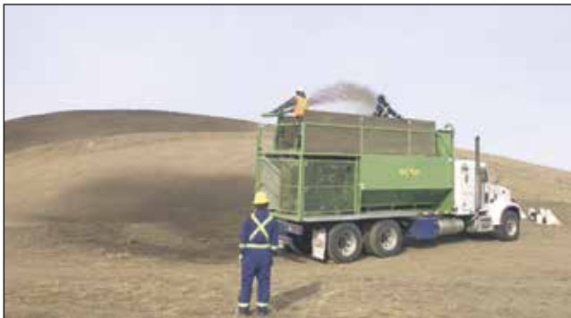
In some areas, seed was applied wet, with a tackifier to adhere to dry slopes.
