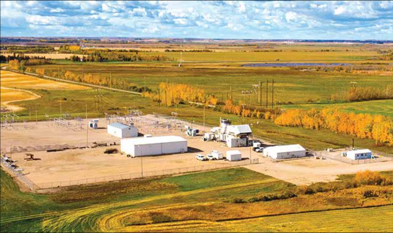
Meadow Lake Power Station – which will soon be replaced. SASKPOWER PHOTO
