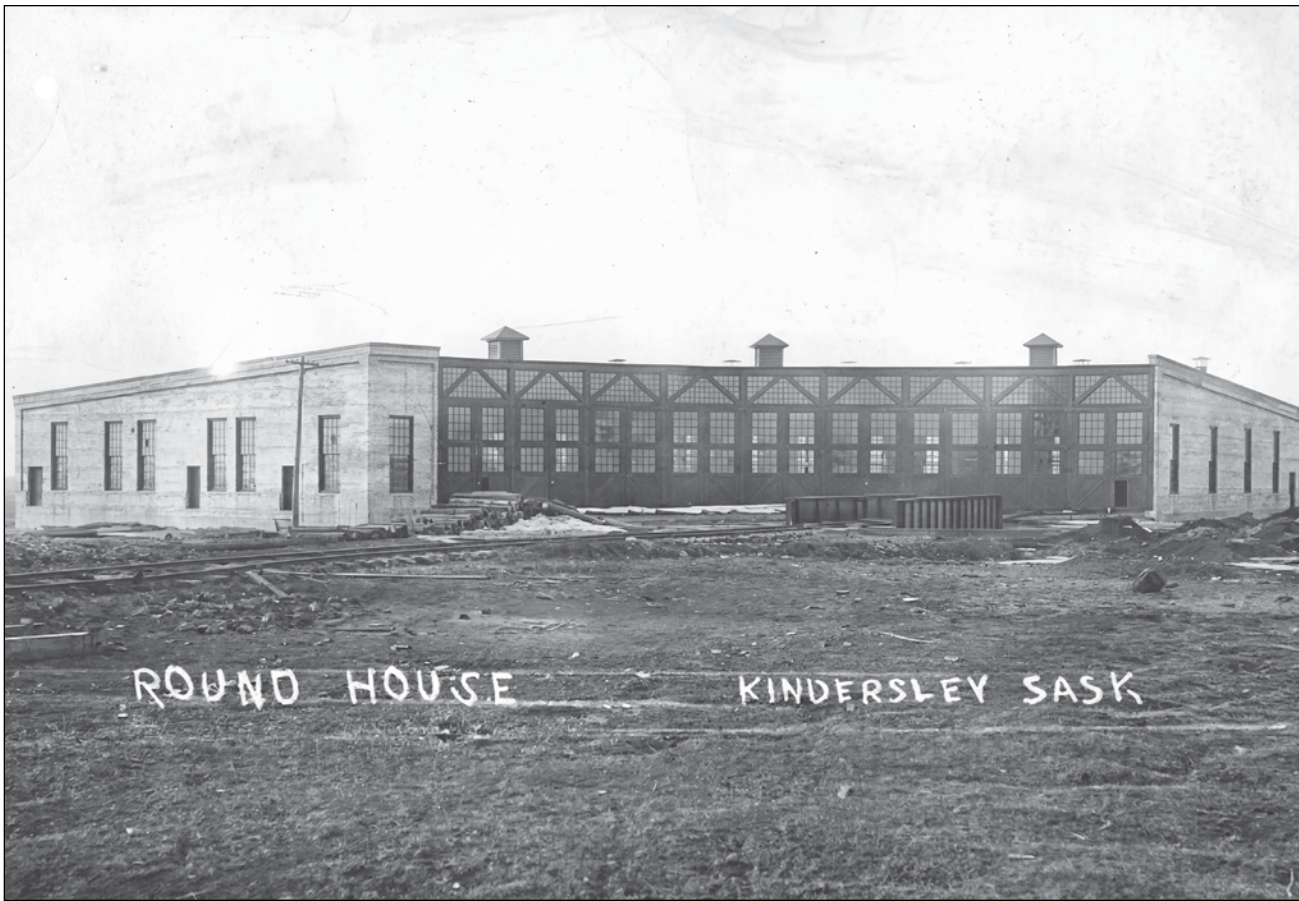
Kindersley's roundhouse in 1922. PHOTO HISTORIC SASKATCHEWAN
