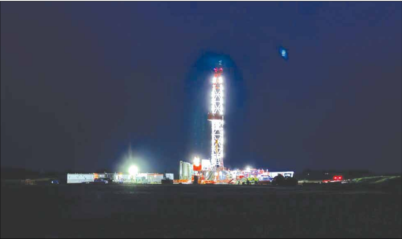
A Betts Drilling rig near Glen Ewen on June 21, 2026. PHOTO BY BRIAN ZINCHUK
