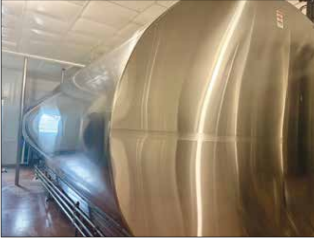
MILK STORAGE: Milk from the colony's dairy herd is cooled and stored in a large stainless steel tank before being hauled to Saskatoon twice a week.
