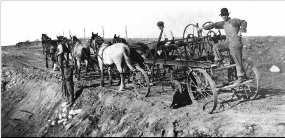
ROAD CONSTRUCTION IN THE EARLY 1900S. It's road construction season on the prairies, with signs posted and traffic slowing down as the work continues. However today's road construction can't compare to road construction that took place in the early 1900s. It was a very slow, tedious and labour intensive endeavour.
