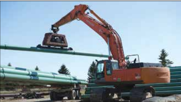
On Sept. 12, 2012, Enbridge was building its Bakken Expansion Project, now Line 26. That project would have figured heavily into its second phase of its Mainline Optimization Project, now on indefinite hold. This photo was east of Redvers. Photo by Brian Zinchuk
