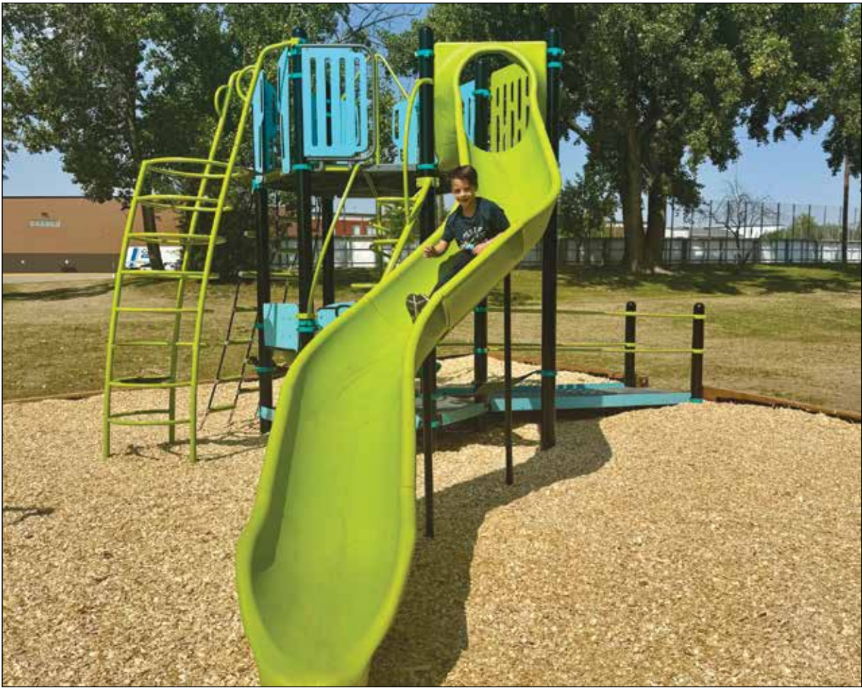
Fresh equipment, instant approval. McGowan Park in Kindersley is partway through a playground overhaul, with the old equipment removed and new pieces going in over the past few weeks. The new slide is already getting a workout. PHOTO BY JOAN JANZEN
