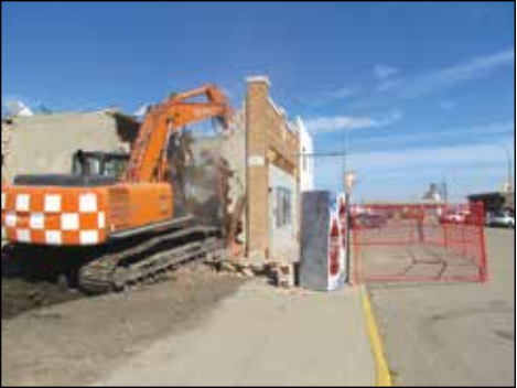
A CENTURY COMES DOWN. An excavator from Adrian’s Demolition of Southey works through the front of the Great West Café on the morning of August 19. The first cut was made at 8:30 a.m. Within 15 minutes of the second cut, the building was rubble.
