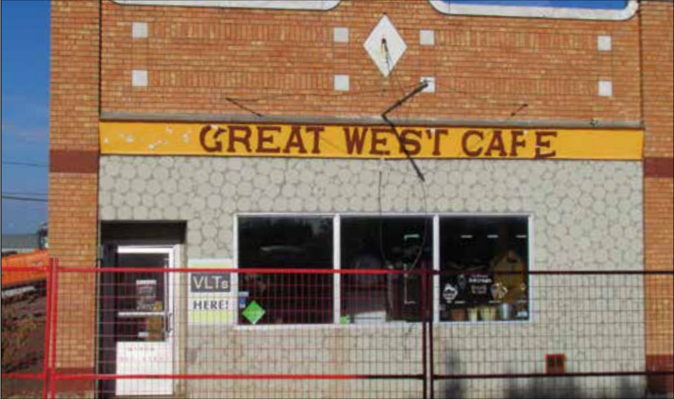
LAST LIGHT ON A LANDMARK. The morning sun catches the Great West Café sign on Eston’s Main Street on August 19, hours before demolition crews began taking down the building. Mrs. Bill Graham opened a café and butcher shop on the site in 1914.
