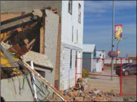
NOTHING LEFT BUT THE FLOWERS. Hanging baskets and street banners frame what remained of the Great West Café after the façade fell. The building had stood empty for years before the August 19 demolition.
